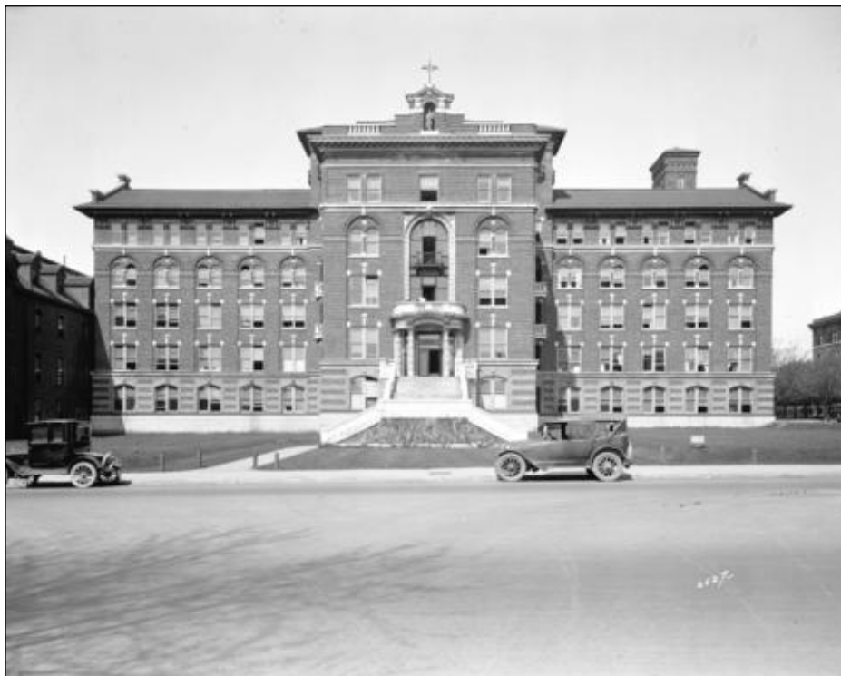
St. Paul's Hospital, Vancouver in 1935 Vancouver City Archives AM54-S4: BU N437.2
